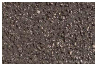
Fig. 2.3 Open graded friction course surface
