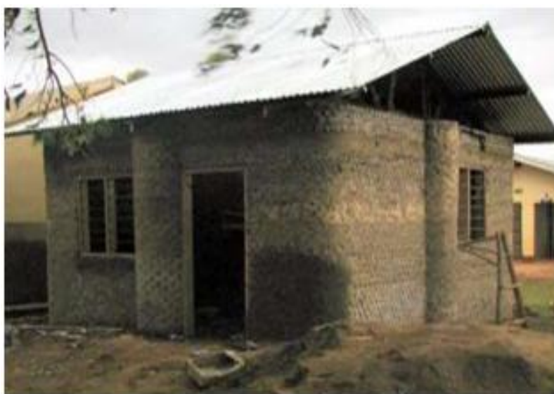
Figure 3 First bottle house construction.
