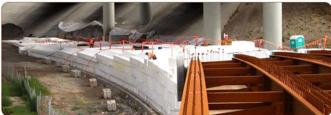
Figure2:Geofoam Utilized as Projection Backfill EPS
