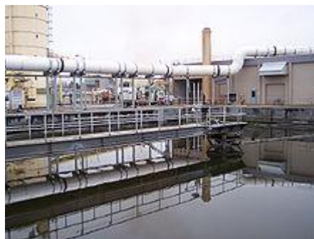
Rectangular primary settling tanks at a sewage treatment plant
