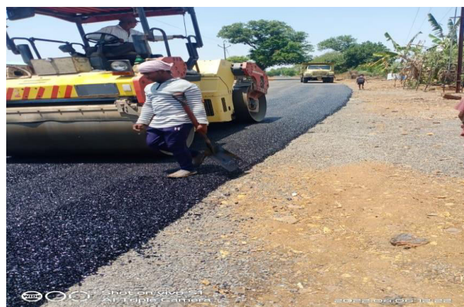
Fig 3- Preparation and placing of Premix.
