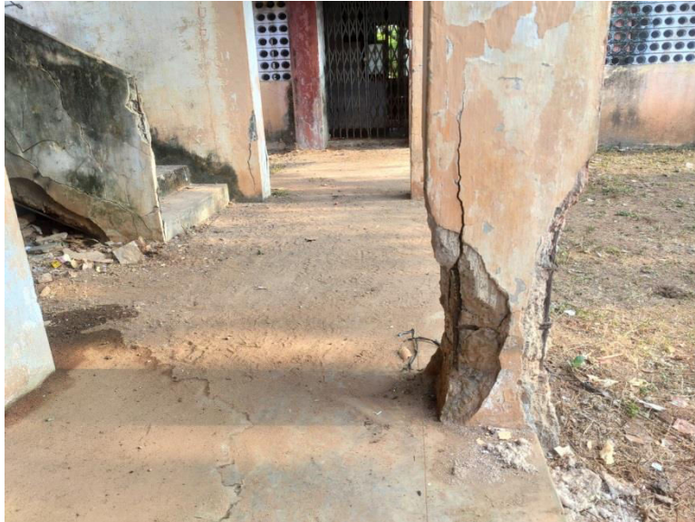
Fig-1 Corrosion crack in column
